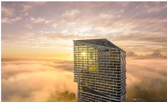
Quay Quarter Tower, Sydney, New South Wales, Australia.
